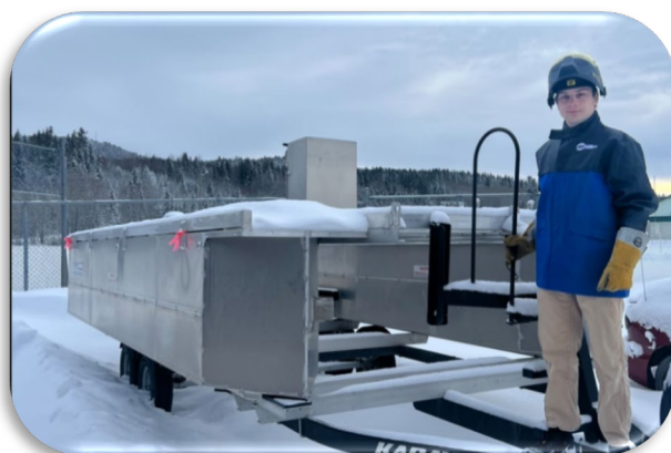
Dan Labatch Free – showing the SFSP under construction
